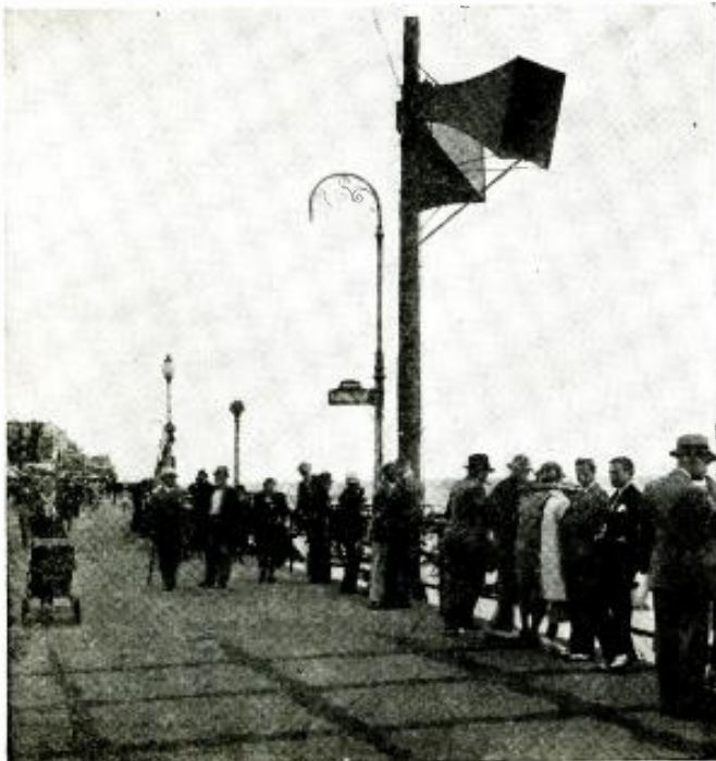
In the view above is illustrated a practical application of the principles discussed by Mr. Denton. This sound system, an installation on the boardwalk, Long Beach, New York, is designed to "address" a promenading public totalling 725,000 each week!
